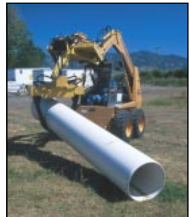
Place pipe in tight angles
